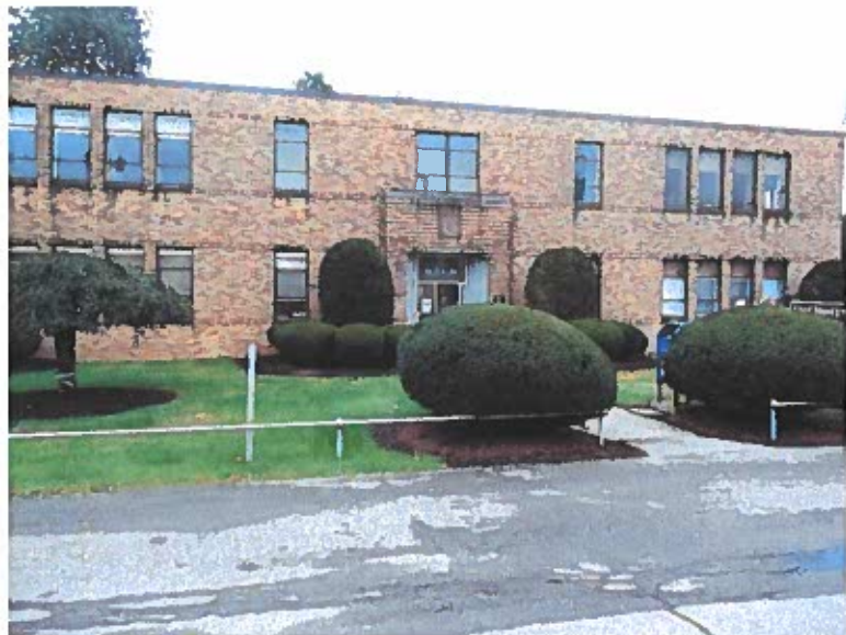
Proposed area in front of building where a designated handicapped parking space will be installed
