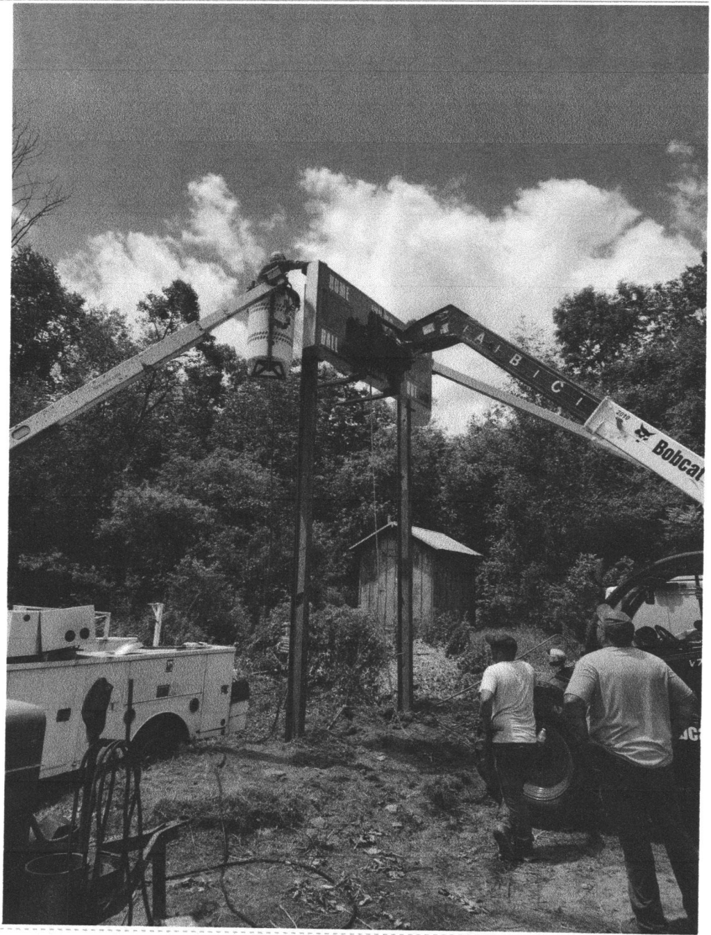
Install of New Scoreboards
