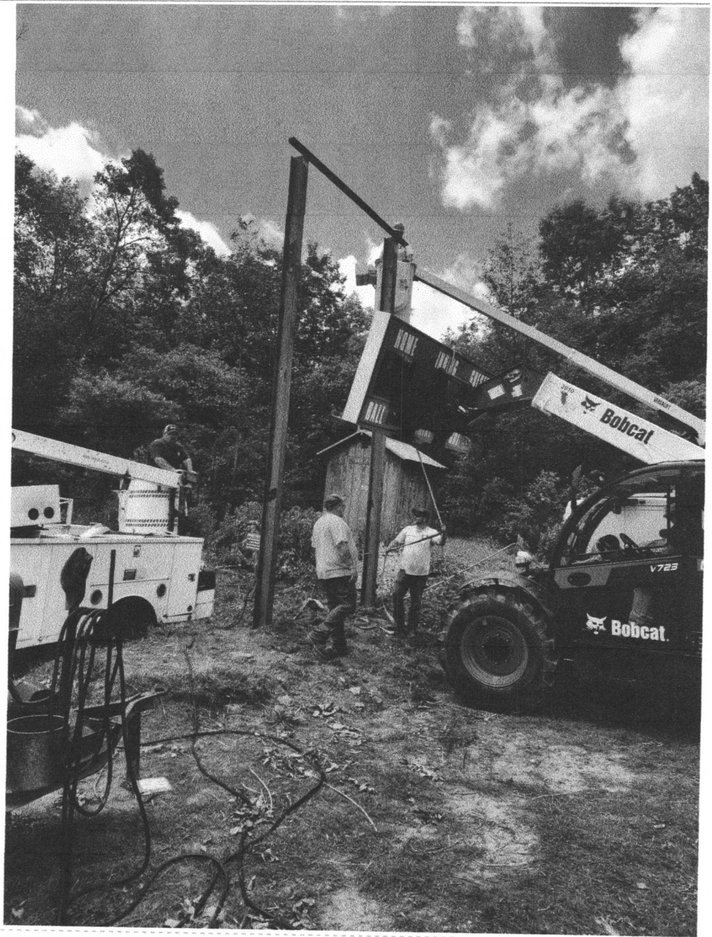
Install of new scoreboards
