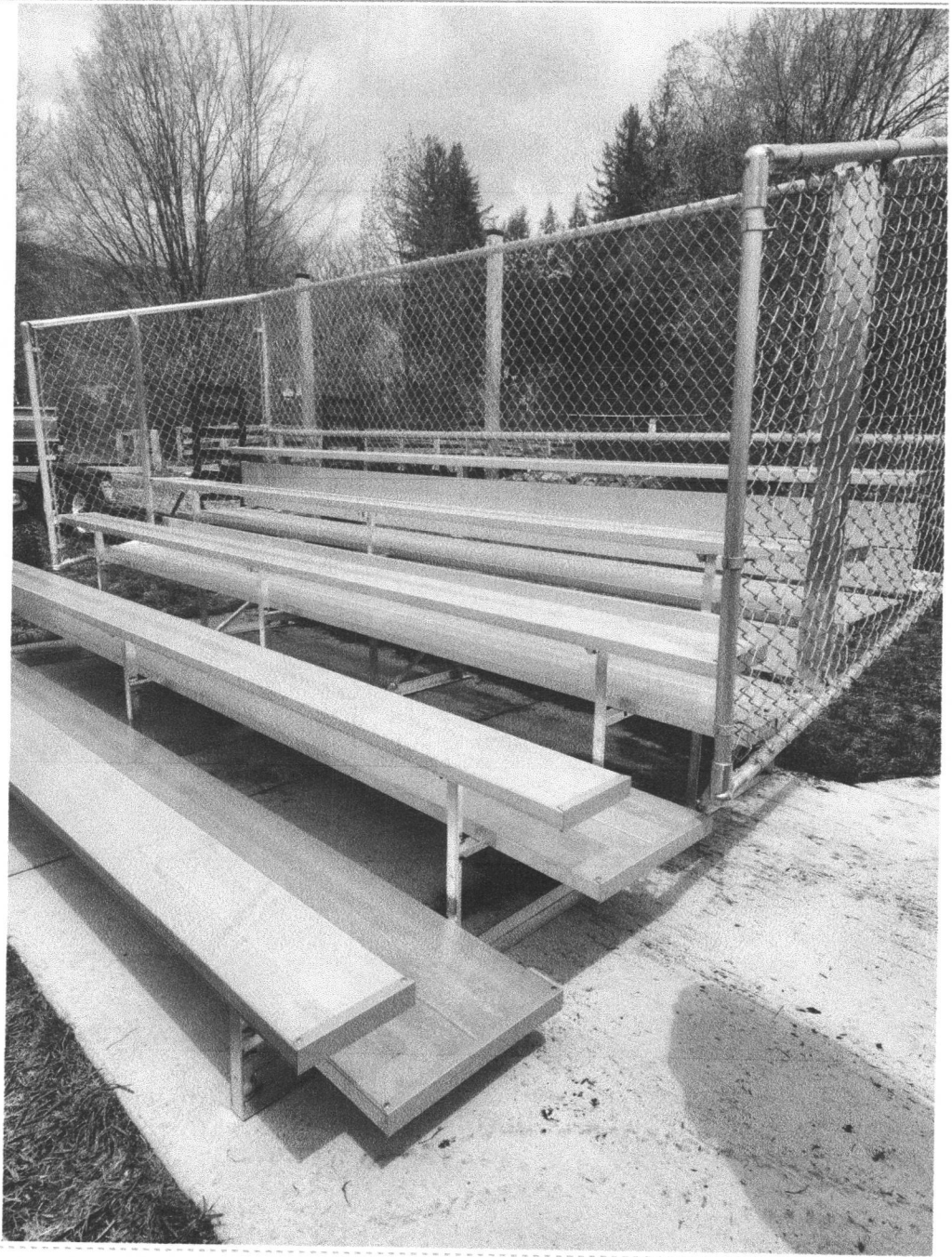
New bleachers built and placed on pads at all baseball flds in Callahan Park.
